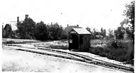
FIG. 2.—WYETH SWITCH, DAFT THIRD-RAIL ROAD, BALTIMORE.
